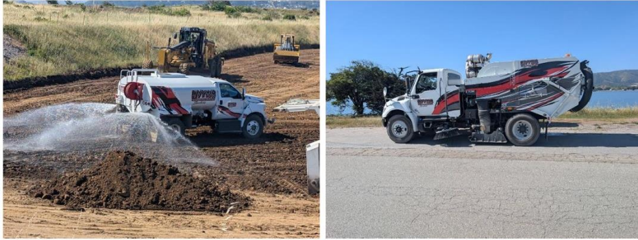
Images above. Best practices to suppress dust through site watering and cleaning equipment to reduce track out. Left image. Four air monitor locations indicated by yellow pins.
