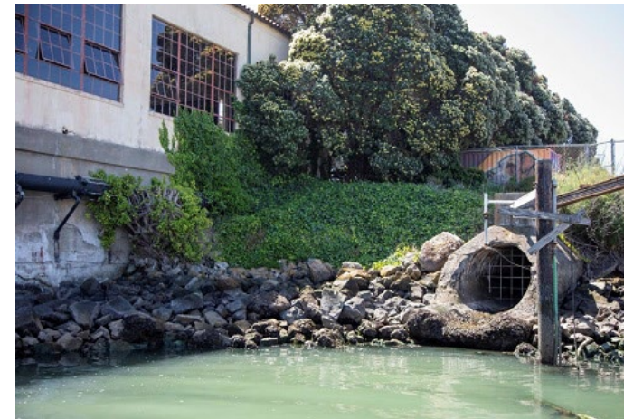
Image left. Existing outfall, Laguna Street, San Francisco
