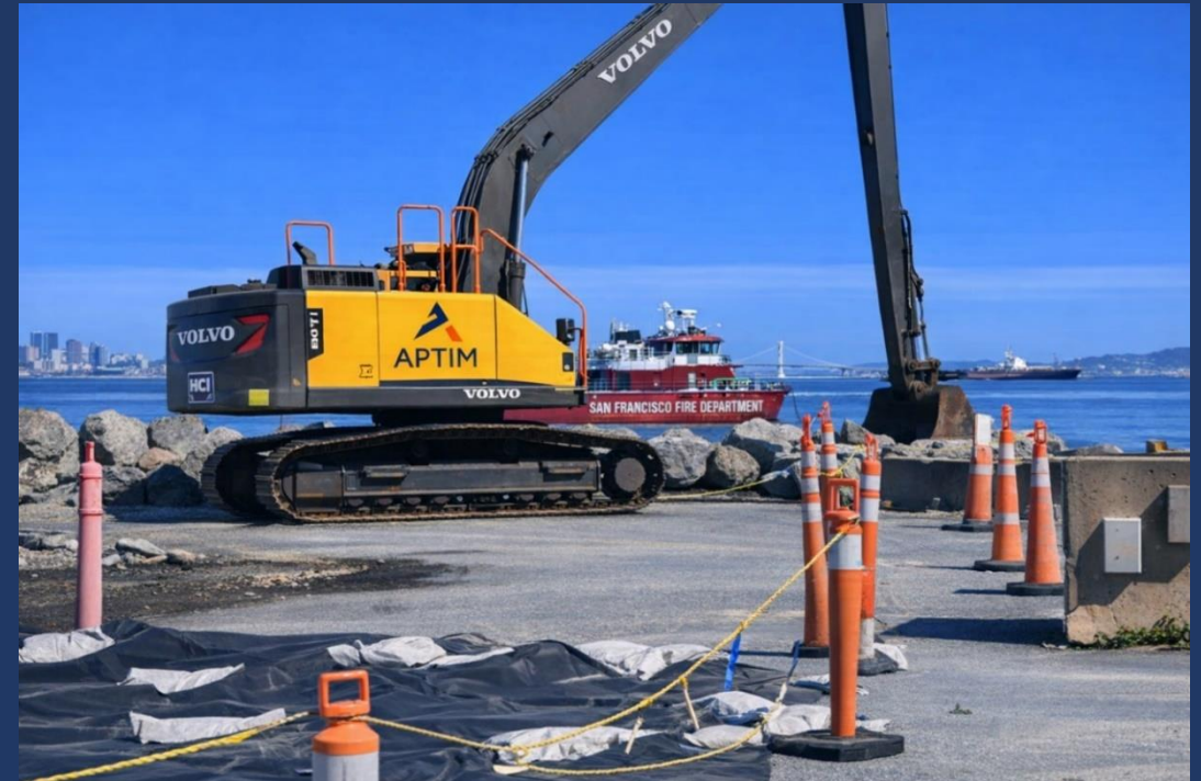
APTIM performing Parcel C Dry Dock Repair
