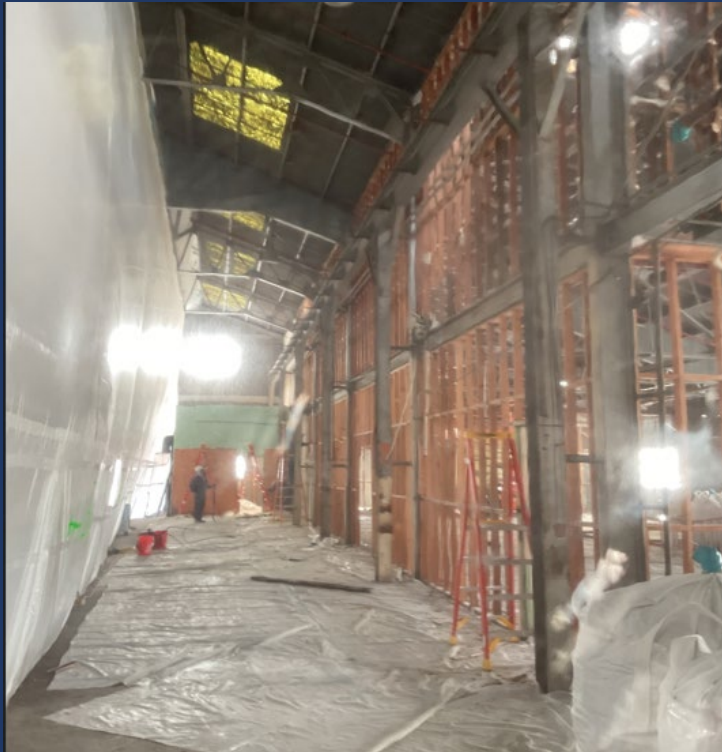
BLDG 366 Interior Work
