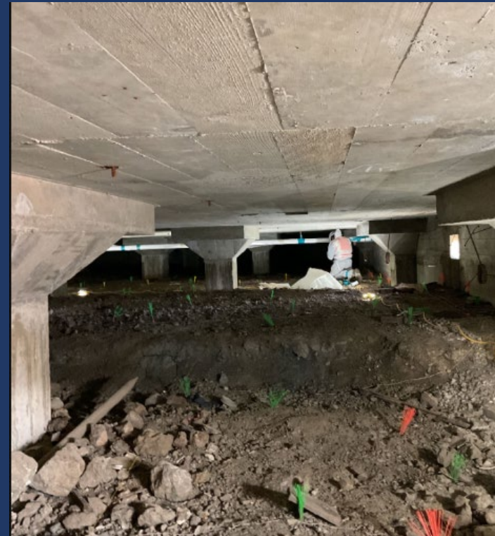
BLDG 351A Crawl Space Abatement
