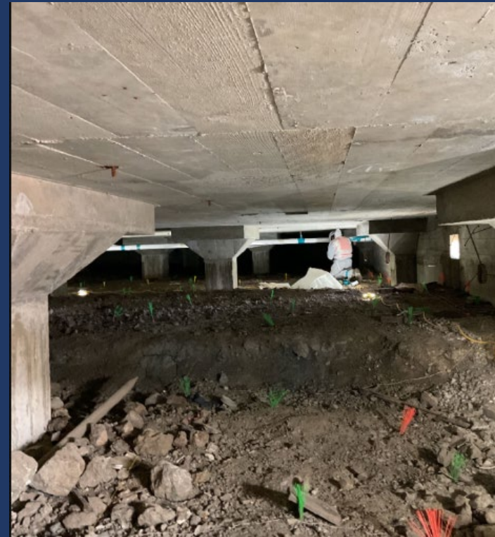
BLDG 351A Crawl Space Abatement
