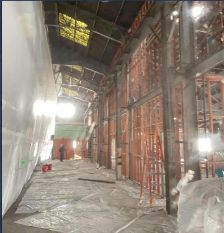
BLDG 366 Interior Work
