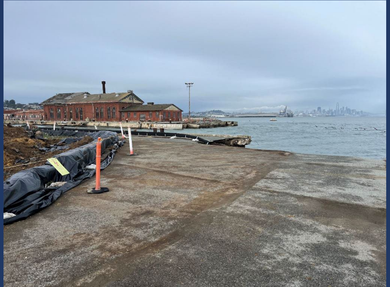
Relocated RSY pad, moved away from eroded area
