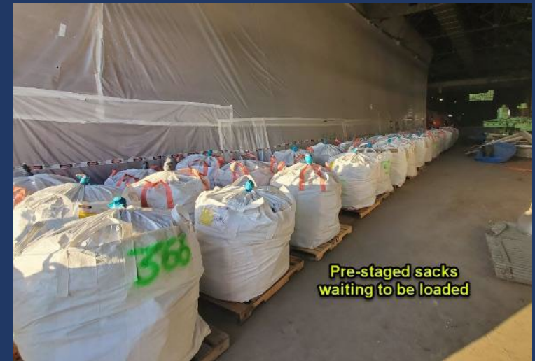
Loading of asbestos pipe
