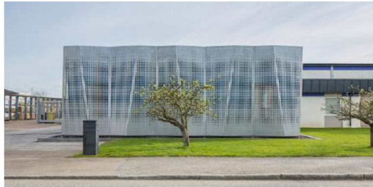
OFFICE EXTENSION, JOHAN SUNDBERG ARKITEKTUR, LUND, SWEDEN
