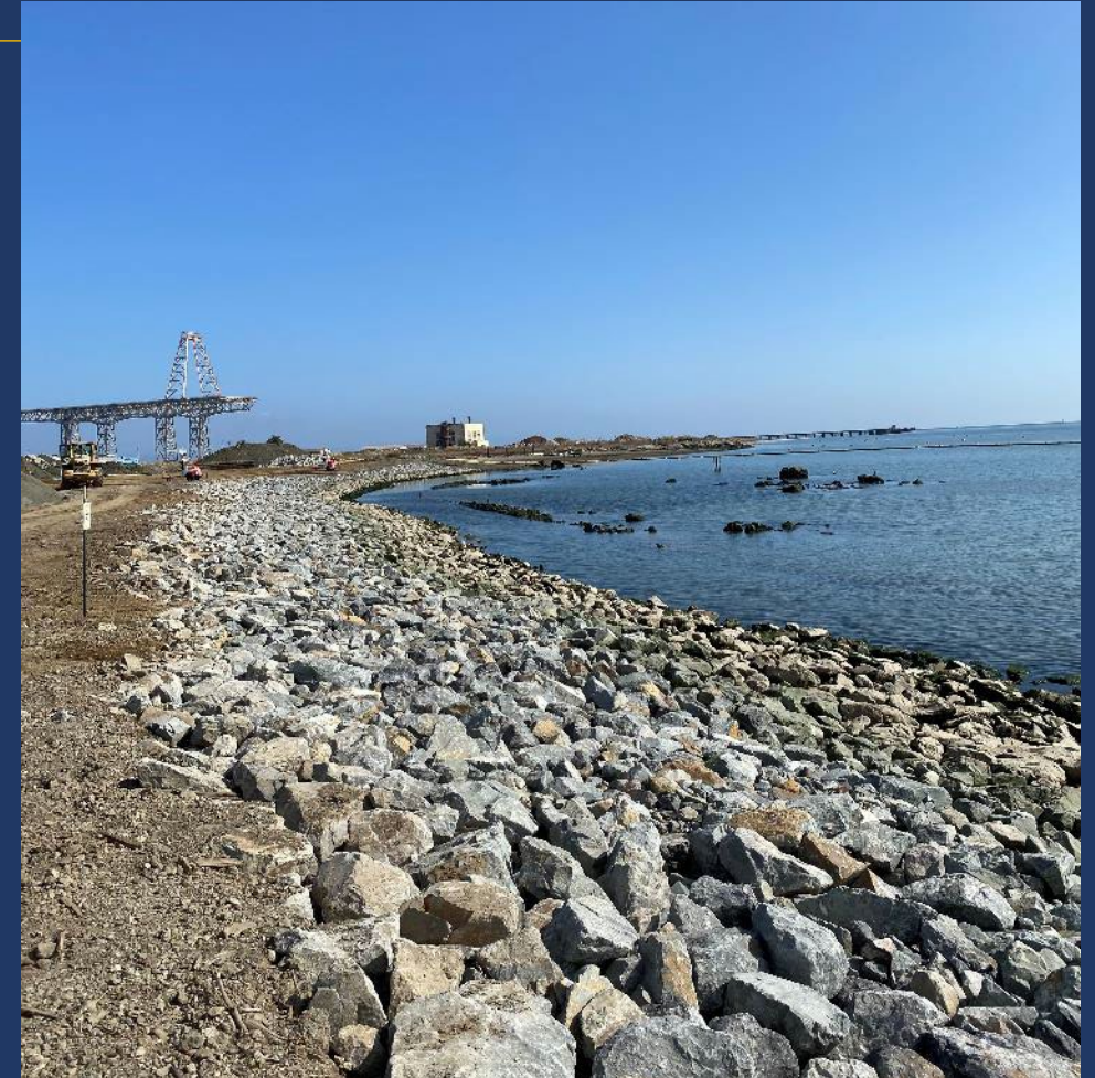
Rock revetments have been placed along portions of the Parcel E shoreline to protect the San Francisco Bay
