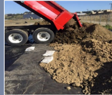
Excavated soil on radiological screening yard (RSY) pad
