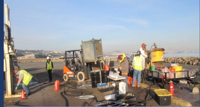
Mixing compound before injection
