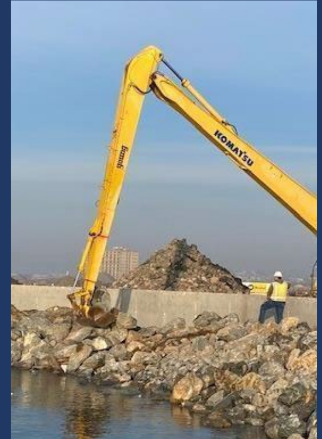
A 27-foot-wide rock “revetment” and a 3-foot-high sea wall protect 550 feet of Parcel E shoreline
