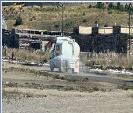
Wetting of haul road to reduce dust
