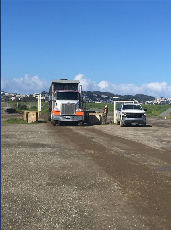
Trucks passed through radiological screening portal when exiting site
