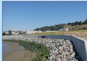
A rock "revetment" extends up to 9 feet above mean sea level to provide a barrier from Bay waters at Parcels E and E-2 shorelines. A 3-foot high concrete sea wall sits above portions of the revetment to limit the impacts from the Bay during extreme weather events.
