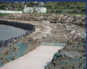
Nearshore "slurry walls" limit groundwater flow off of Parcels E and E-2, protecting the shoreline and reducing erosion
