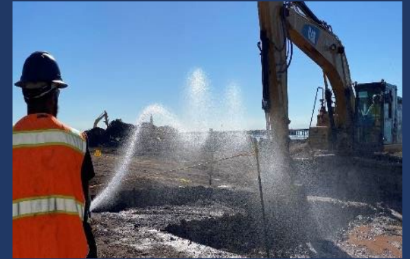
Example of dust suppression best practices used during excavation and demolition
