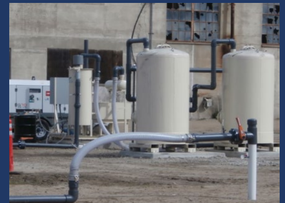
An extraction system removed vapors from soil
