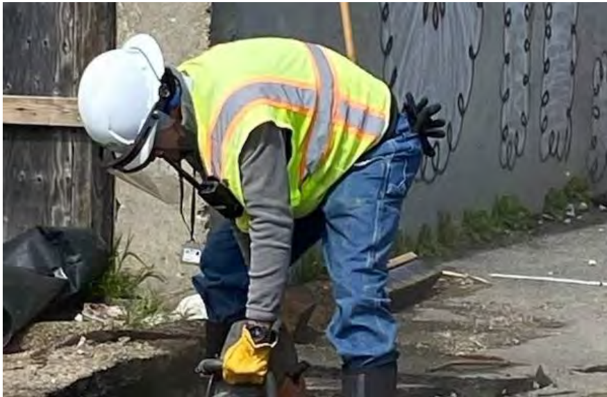
Preparatory Saw Cutting at Trench Units
