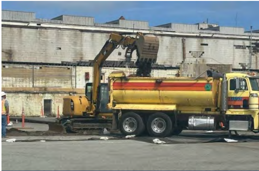
Radiological Excavation and Loading of Trenches
